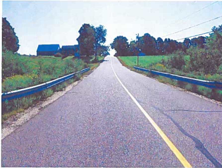
PHOTO 1 Description General roadway east
